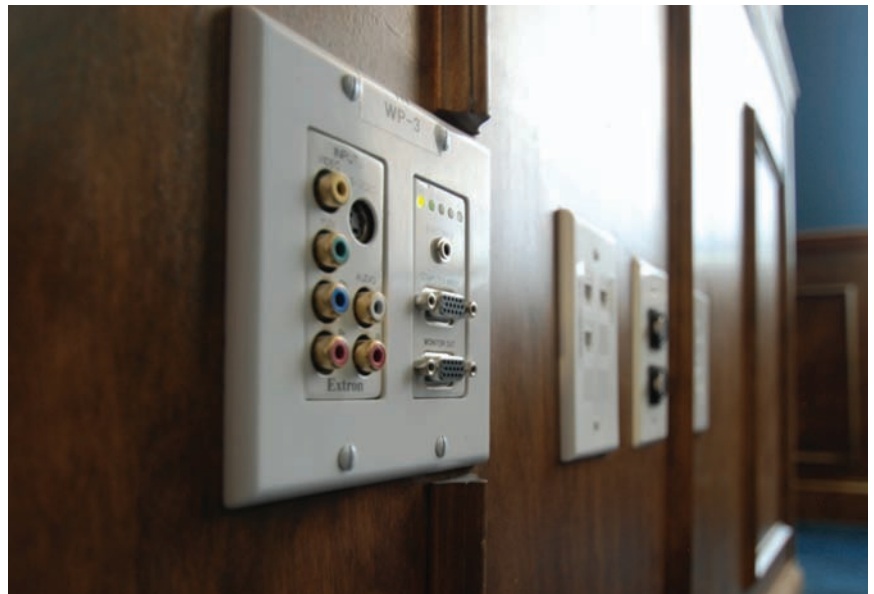
Extron wall plate with component, S-Video, VGA, and audio inputs plus VGA monitor out.
